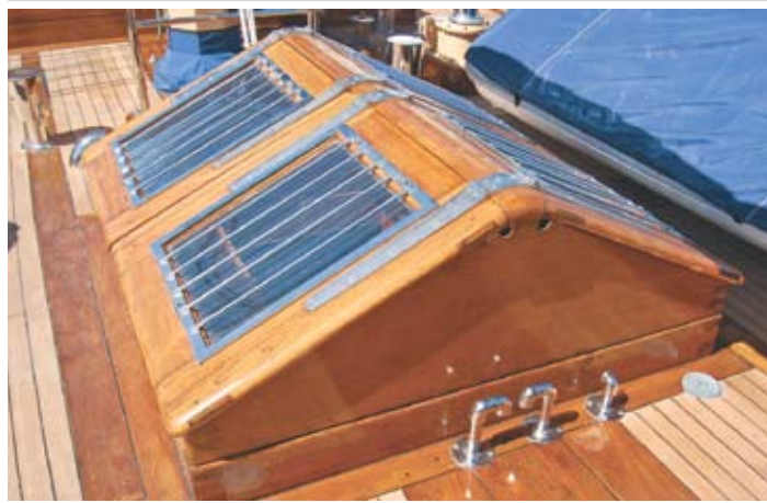
The new deckhouse and hatches were all put together without a single metal fastening. New gratings were made to match the originals.
